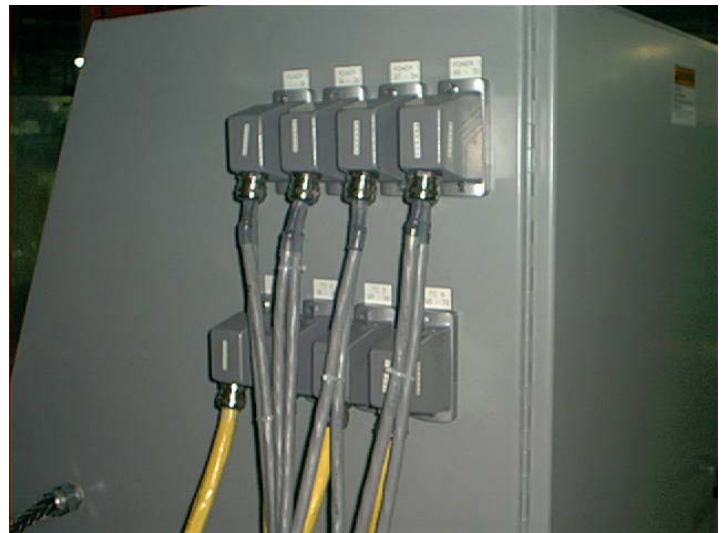
Prefabricated cables installed. 24 zones per cable.
